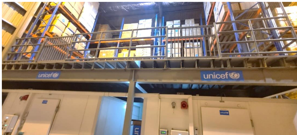
Figure 1 the repaired mezzanine floor in the regional vaccine warehouse ©UNICEF Pacific/CCaloy
